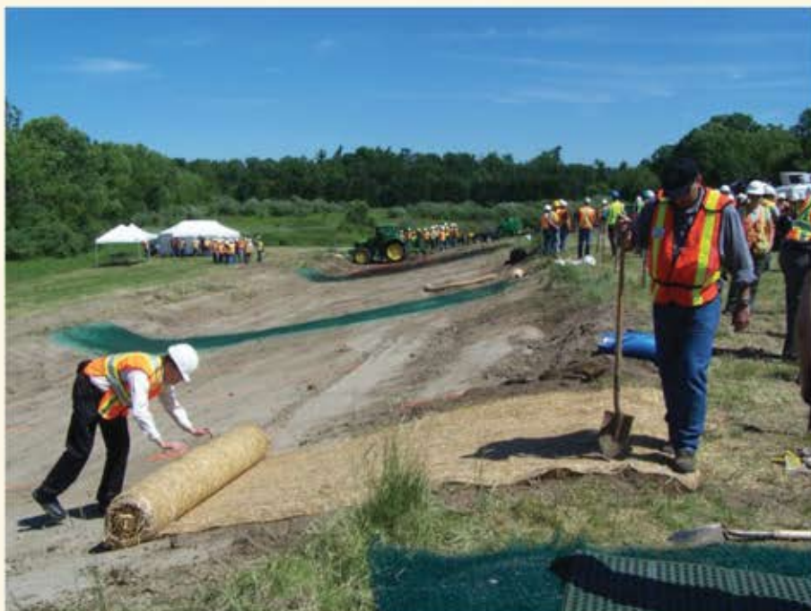
Field day participants work with mats to stabilize a slope.
